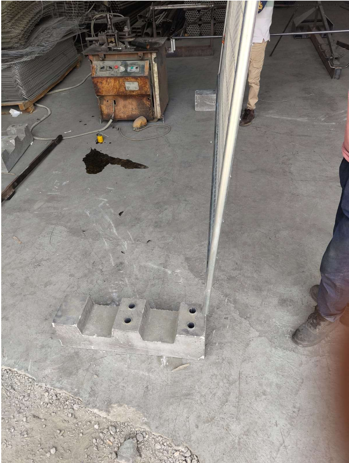
Placing Second side of panel on second footing at 3.5m distance
