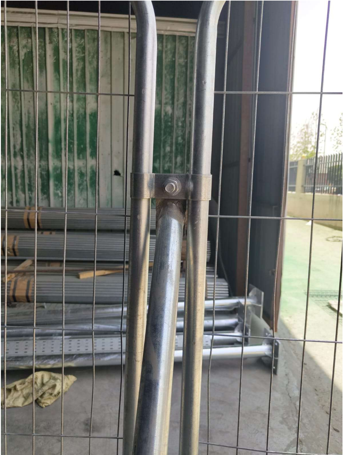
Installing Back support with Galv Clamp and Hex Bolts
