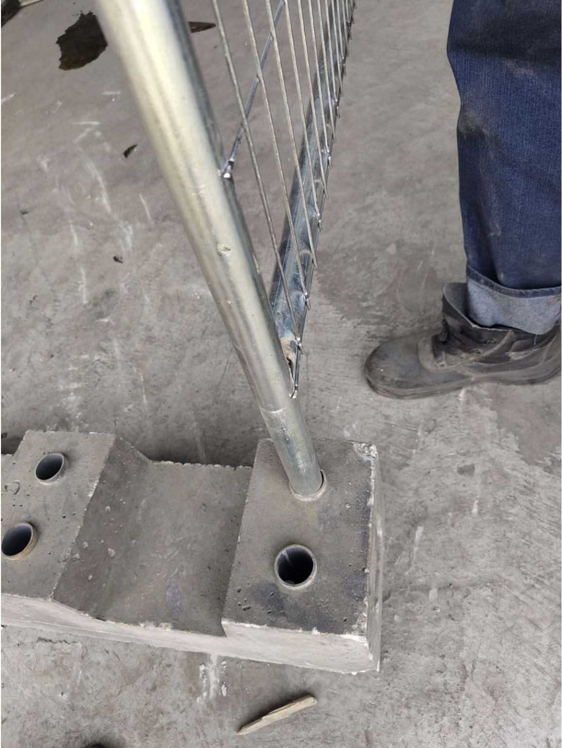
Placing one side of Panel on Concrete Footing
