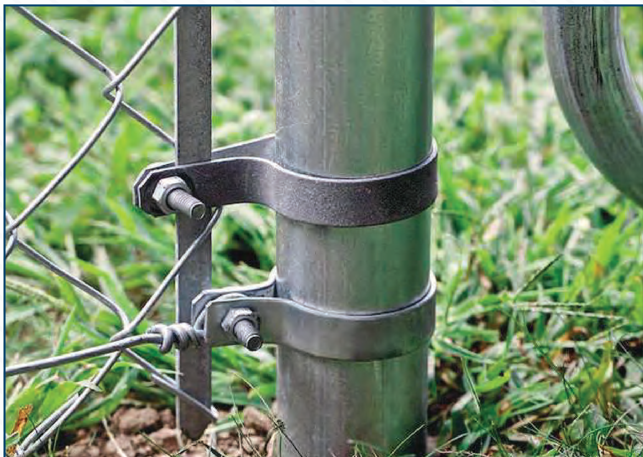
Carriage bolt tighten tension band
