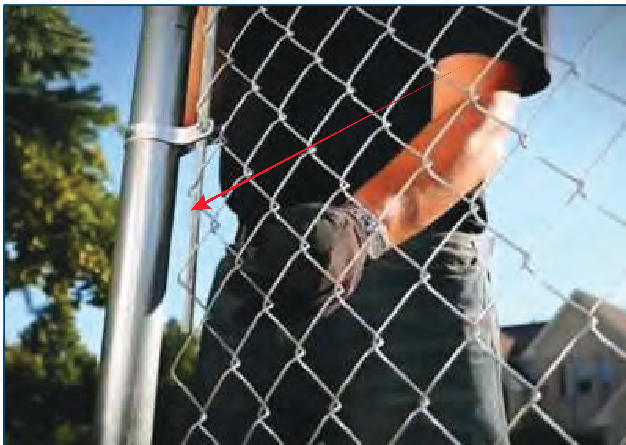
Tension bar attaches chain link panel
