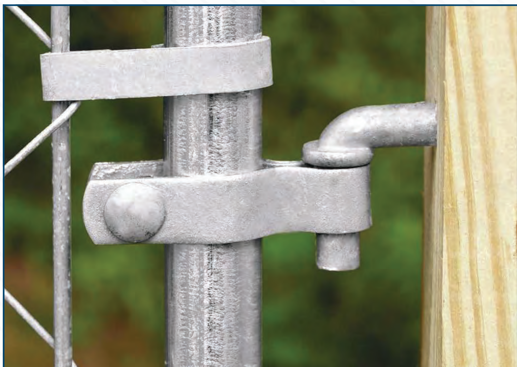
J-bolt hinge connects post to the wall
