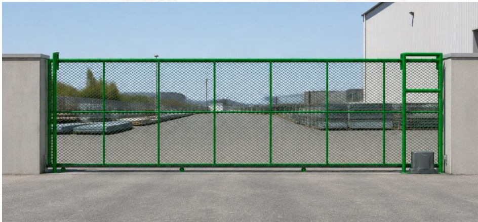
Routine inspection: carriages, track beam, lock, guide roller and finish
